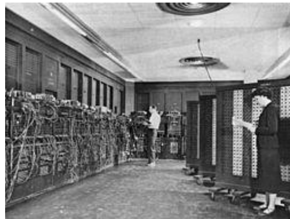
Figure 1. The ENIAC Computer (source Wikipedia) contains 70.000 resistors.
